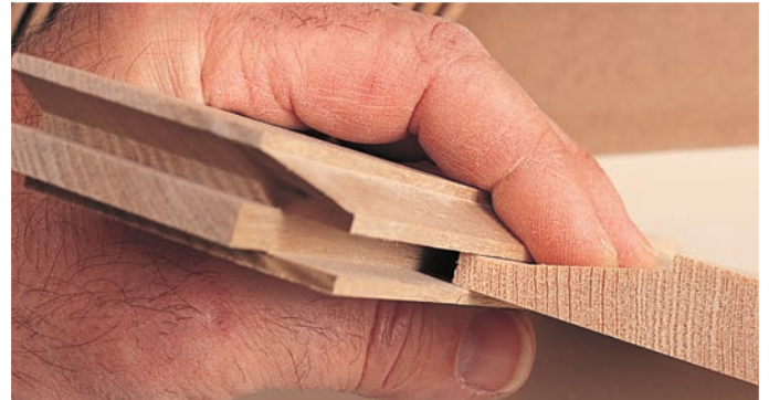
The proof of your setup is in the fit of the panel to its groove in the frame. Make a cut on a sample of the panel stock and fit it to an actual frame member. The ideal is a snug press fit.
